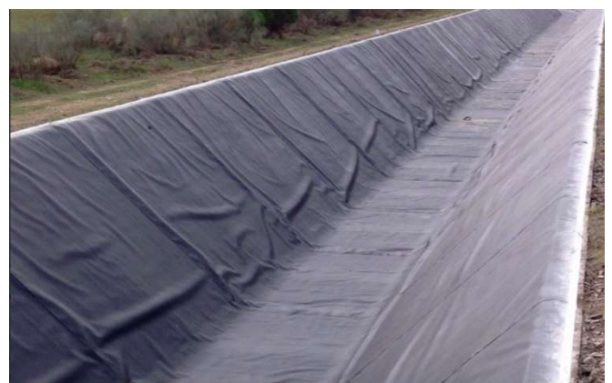
Figure 6. Laying a geomembrane along a canal in Spain [23]
