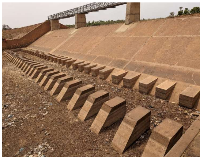
Figure 3. Zongo Dam during low water period
