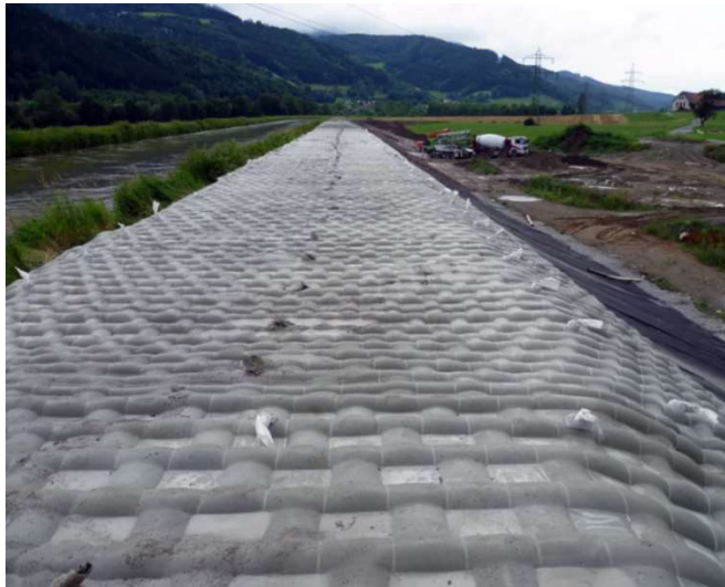
Figure 7. A dike strengthened with geotextiles [24]
