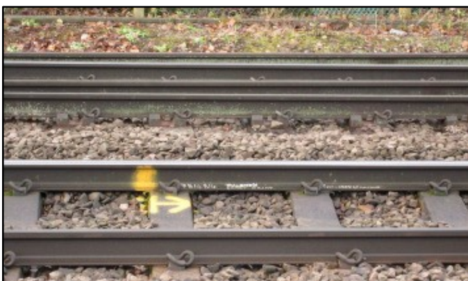
Fig. 4. Continuous welded rail (Jones & Ashby, 2019b)
