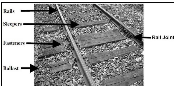
Fig. 3. Traditional railway track with joints
