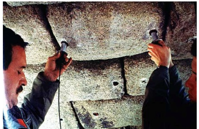
Fig. 15. Auscultation of the ultrasonic transmission speed in the ashlars of the Roman Aqueduct of Segovia (Jurado, 2007)
