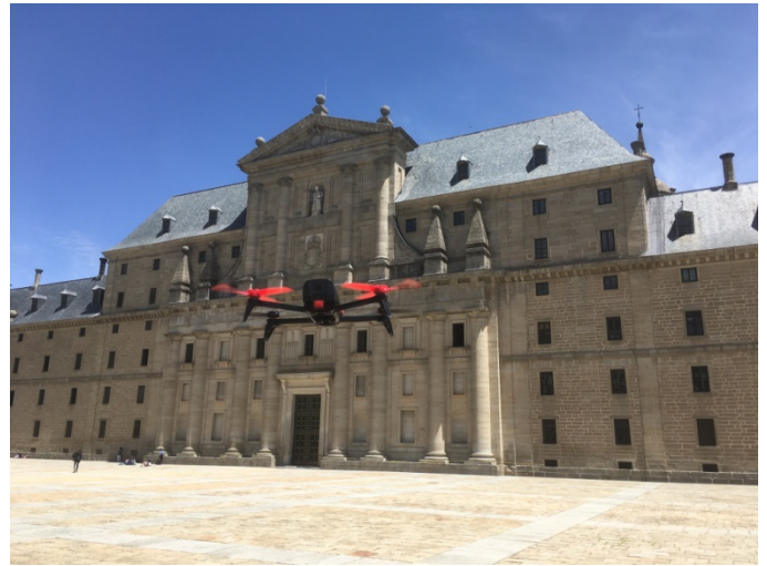
Fig. 2. Quadrotor drone ready to take off, for an inspection on the main facade of the Monastery of El Escorial, Spain (photo by the author).
