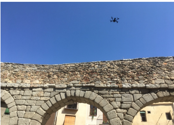
Fig. 1. Quadrotor drone flying over the Roman Aqueduct of Segovia, for inspection (photo by the author)
