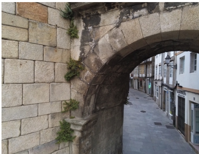
Fig. 10. Flight of a quadcopter drone during the inspection of a singular point of the Roman Wall of Lugo; specifically in the Porta de San Pedro ou Toledana (a) and images captured by the drone (c), where the deterioration of the stone material can be observed (photographs by the author).
