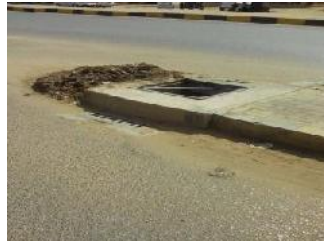
Figure 31. Storm water trenches (34)
