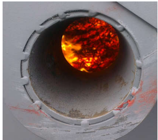
Burning in the combustion chamber observing through the spy hole; Source: Dolina Ltd.
