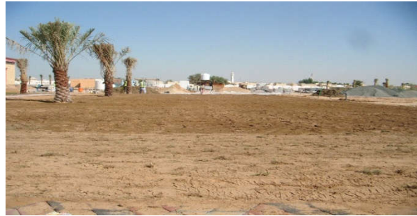
• ABMMRZC mixed with soil and leveled of
