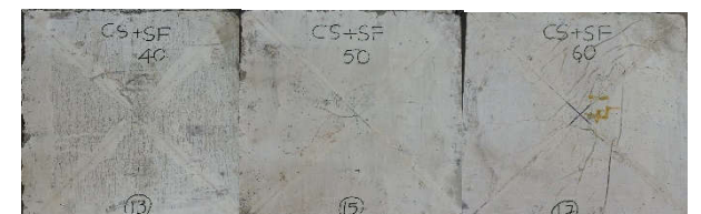
Fig. 4.3. Crack pattern of M60 +SF(40 mm, 50 mm, 60 mm)
