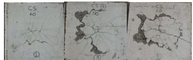
Fig. 4.1. Crack pattern of CS (M60)(40 mm, 50 mm, 60 mm)
