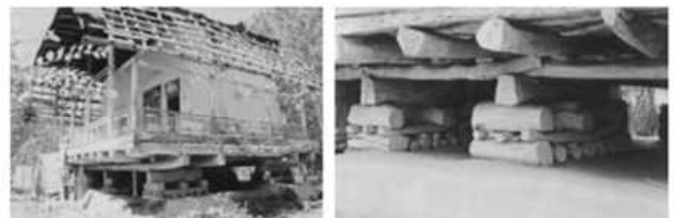
Fig. 3.3. Using the roller system in houses in Lahijan
