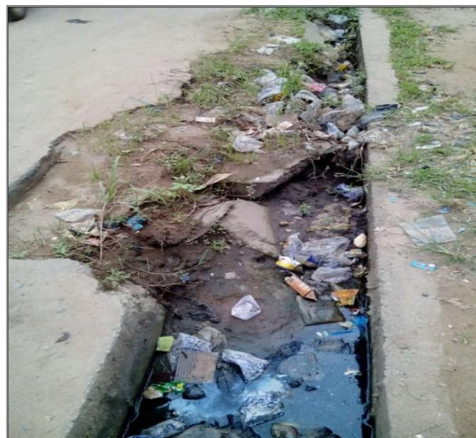
**Figure 3. Drain silted with sludge and refuse**
