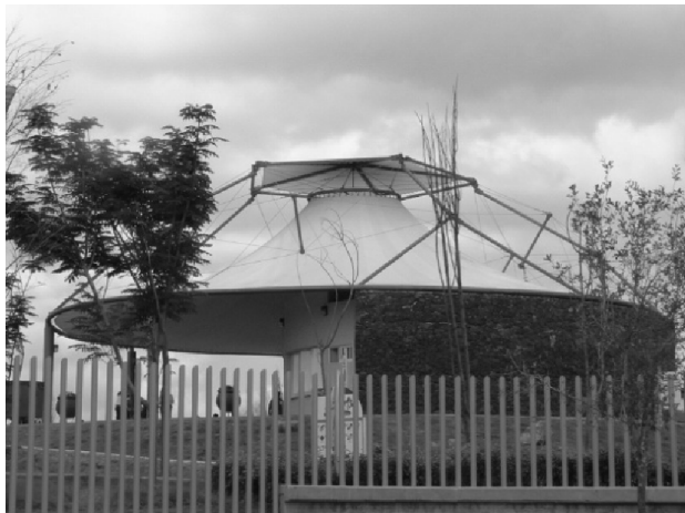
Fig. 1 (a). Prestressed structure coupled to a catenoid membrane. Prototype was built in Alfalfares Park in Queretaro City
